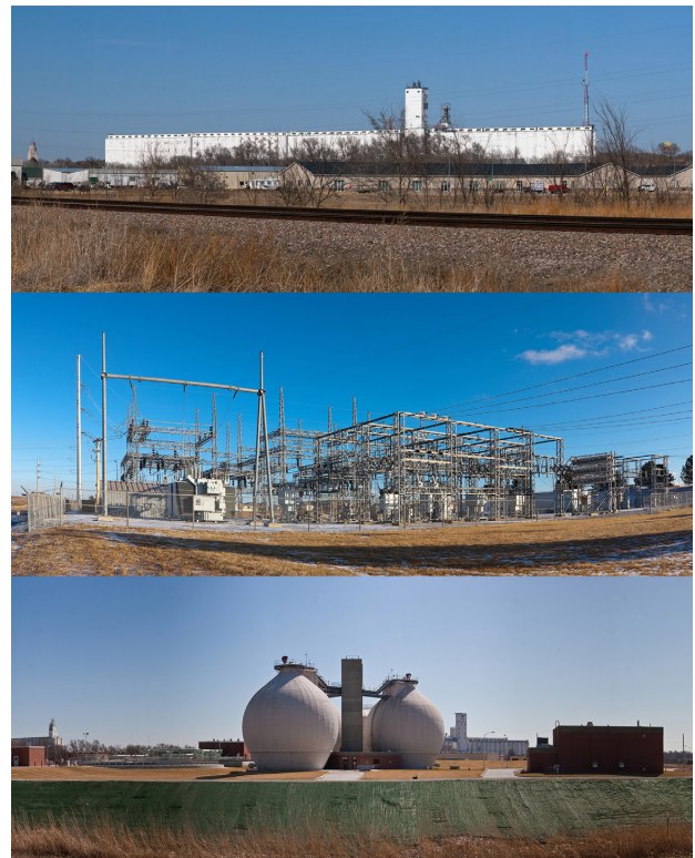
Figure 2. Urban grain elevator, suburban electrical transformer station, and wastewater digesters. Examples of existing infrastructure types in the Lincoln NE viewshed.
